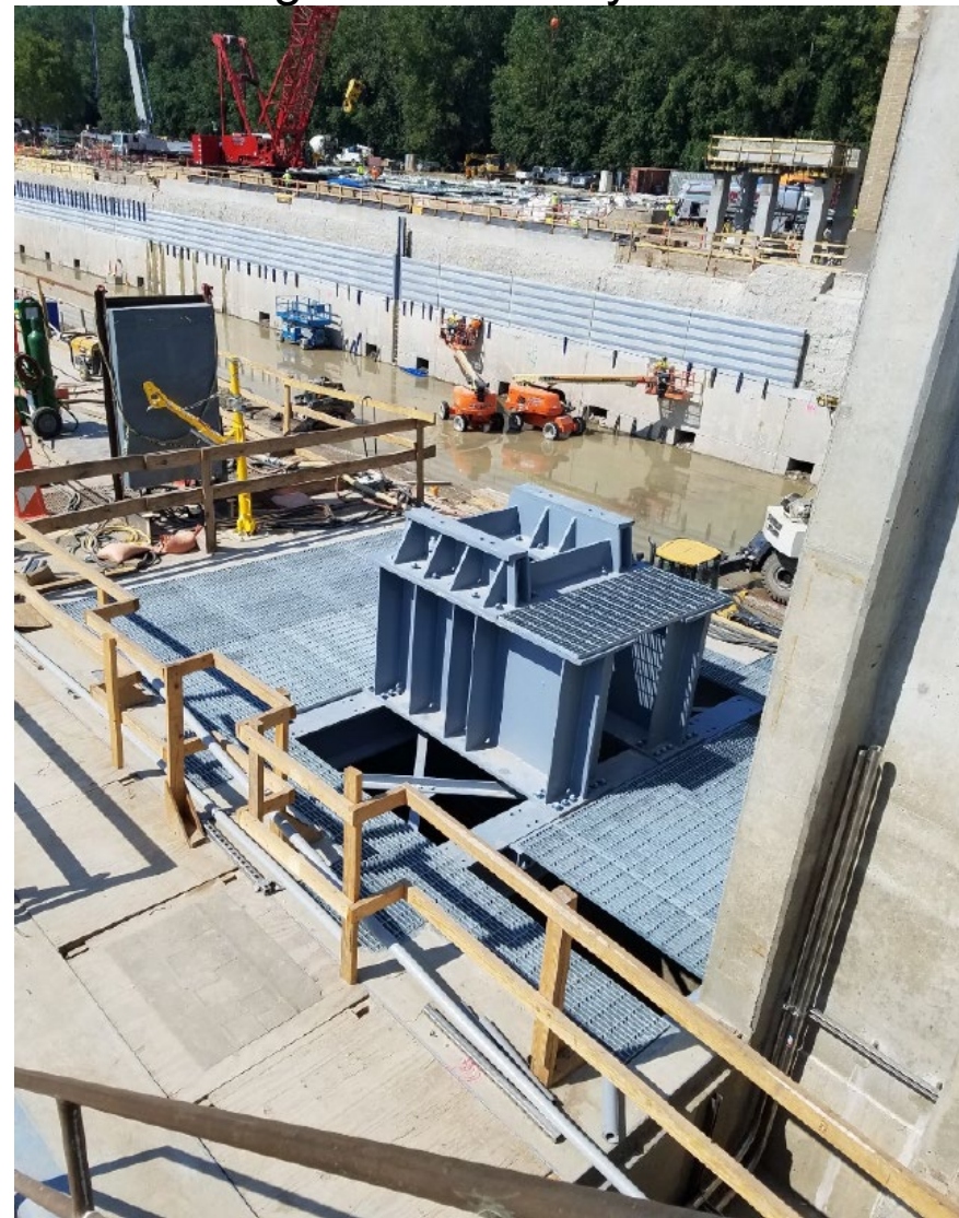
New gate machinery base
