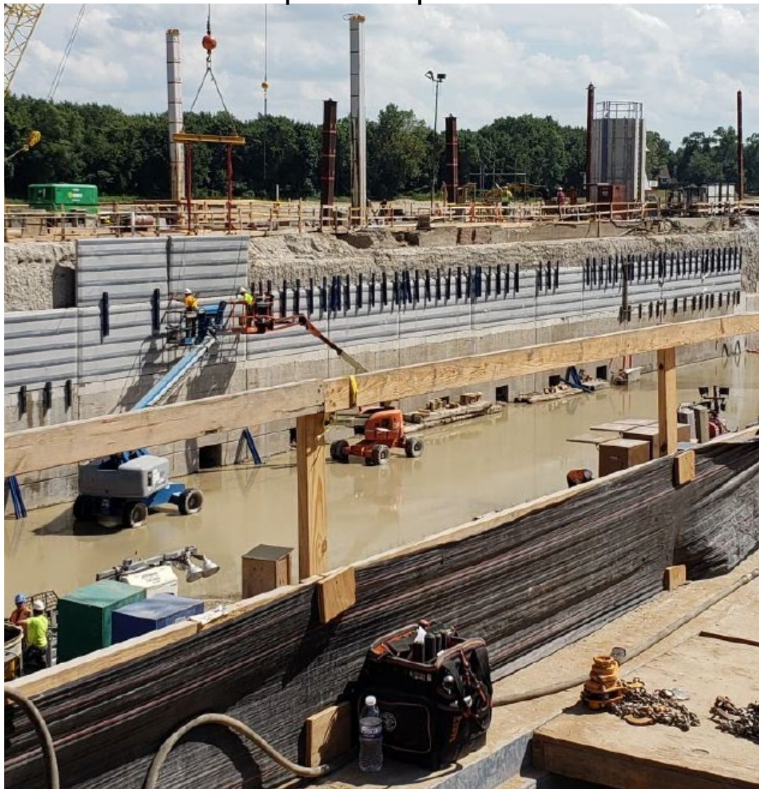
Vertical concrete pre-cast panel installation
