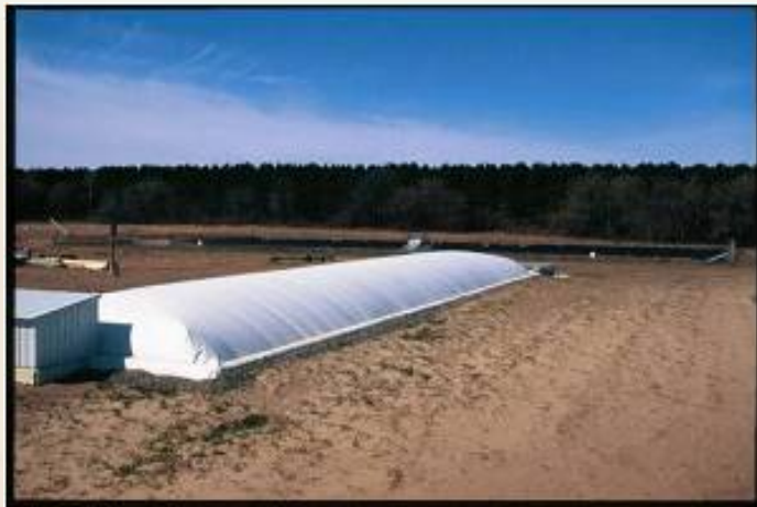
Plug flow digester
