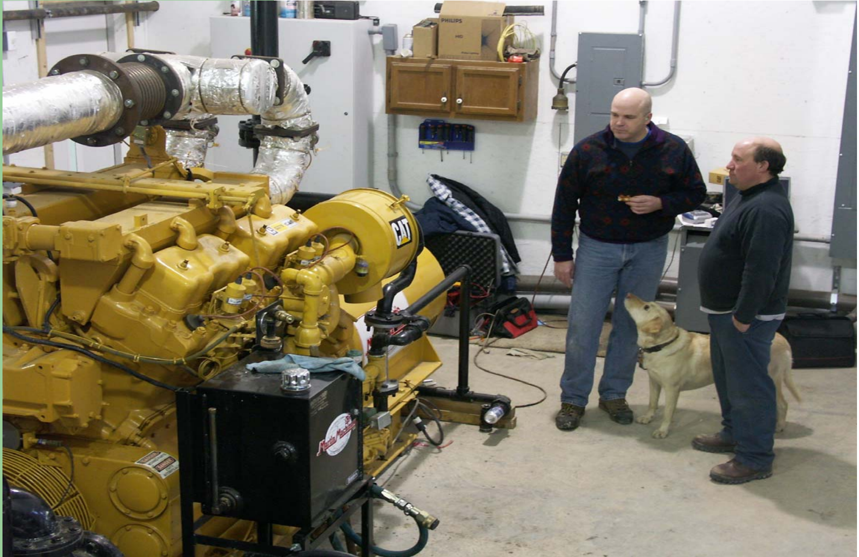
Methane Powered Engine/Generator at Audets
